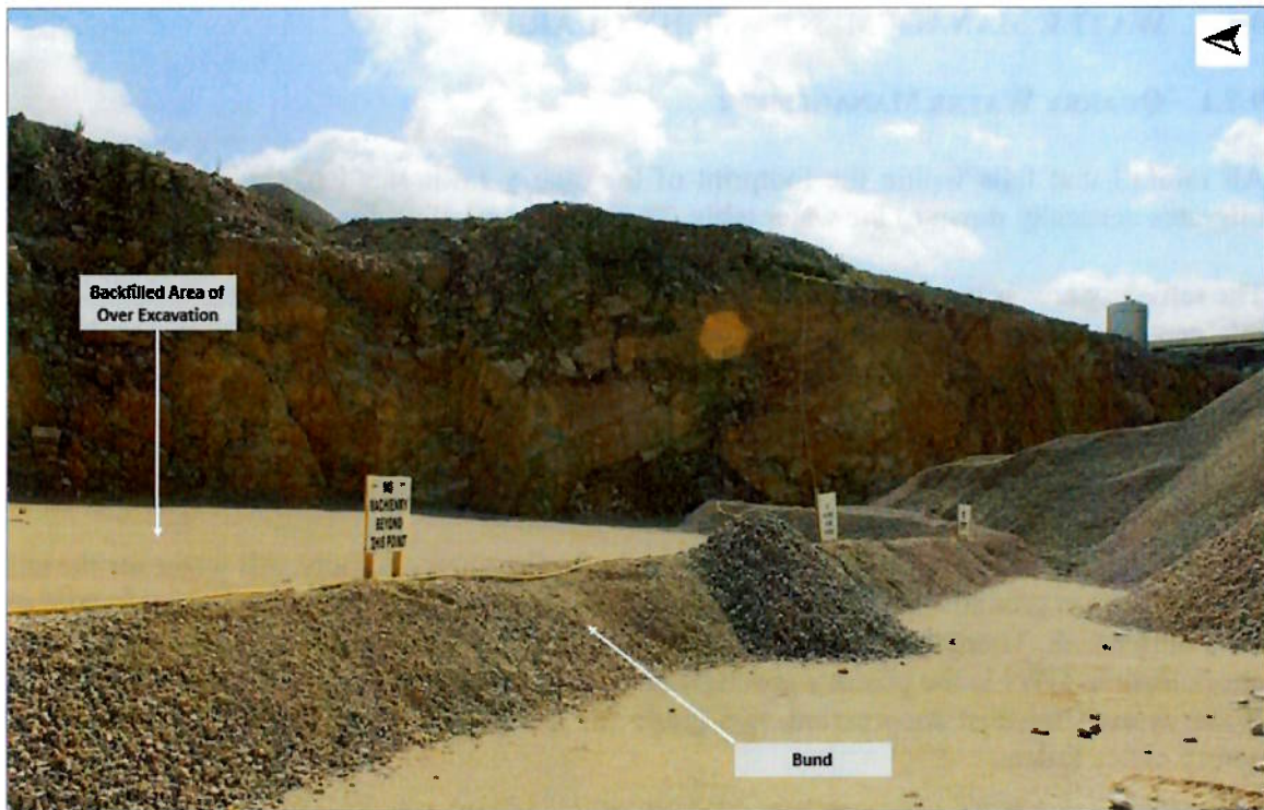
Figure 9.15: Backfilled Area of Historical Over Excavation
